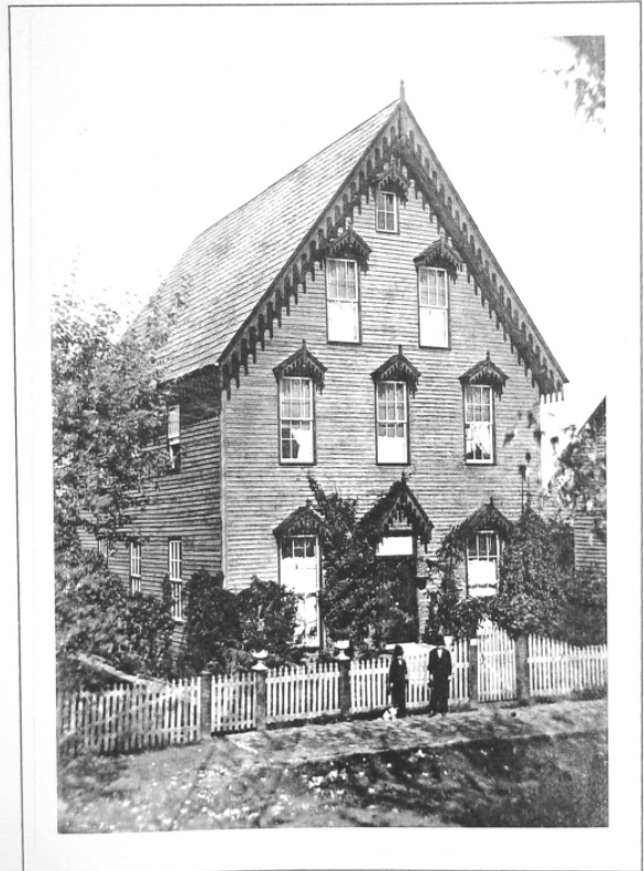
Cottage Institute 1868 -1870 & Woodworth Institute 1869 -1874
